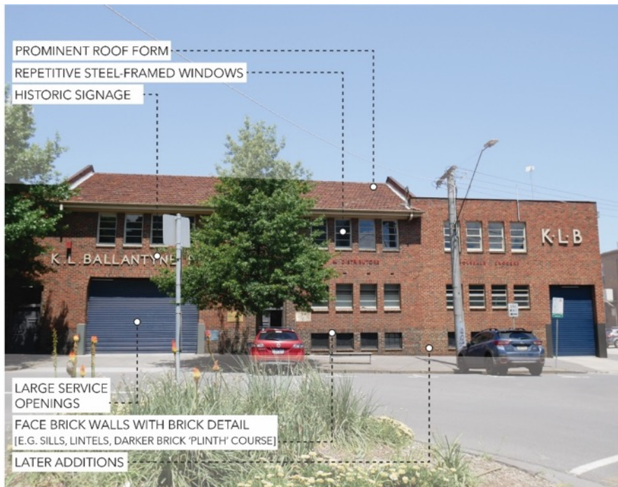
Figure 38. Industrial building typology, with visible roof form, showing typical features.
