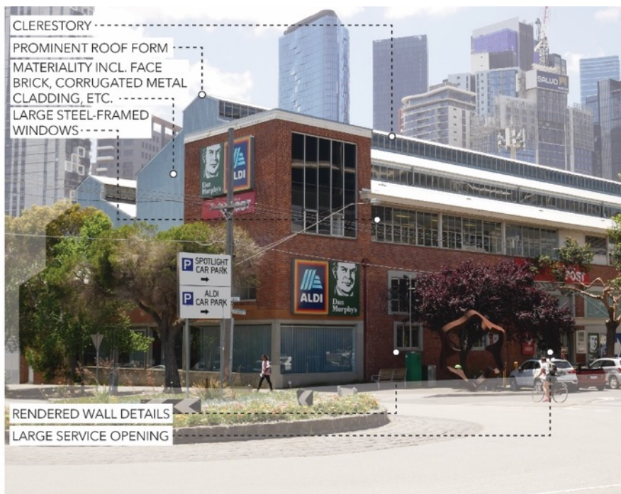
Figure 39. Large industrial building typology, with visible roof form, showing typical features.
