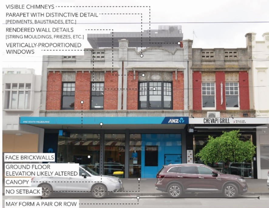
Figure 30. Edwardian shop/residence typology diagram, showing key features. Note: some variation between examples is typical.
