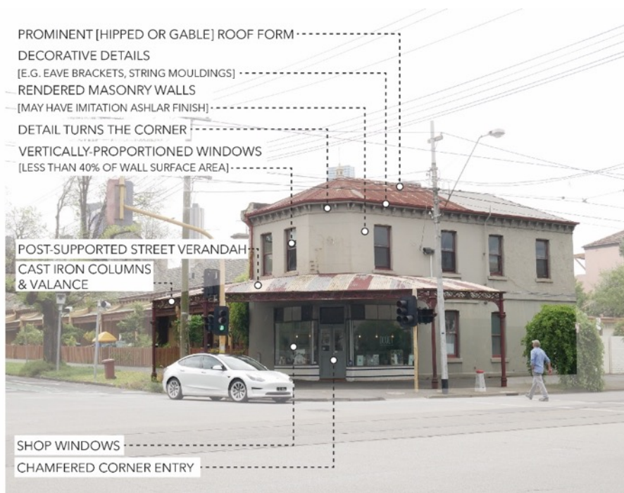
Figure 31. Shop/residence typology as adapted to a corner site, showing typical features.
