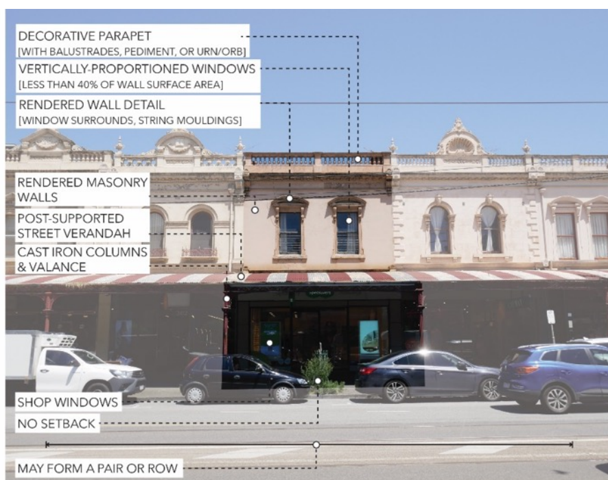
Figure 29. Victorian shop/residence typology diagram, showing key features. Note: some variation between examples is typical. This example is located in Precinct 1 at 300 Clarendon Street, South Melbourne. (VHR H1136)
