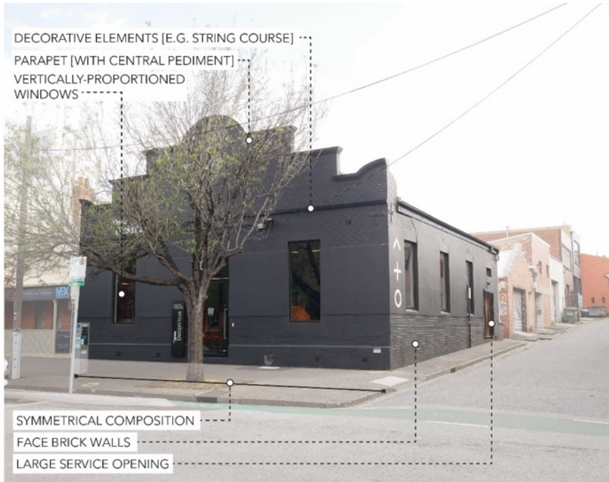
Figure 40. Small industrial building typology, showing typical features.
