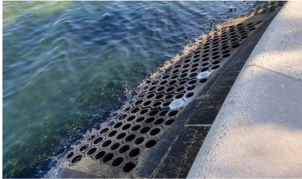
Images left: SeaBee Replacement Beacon Cove, Port Melbourne
