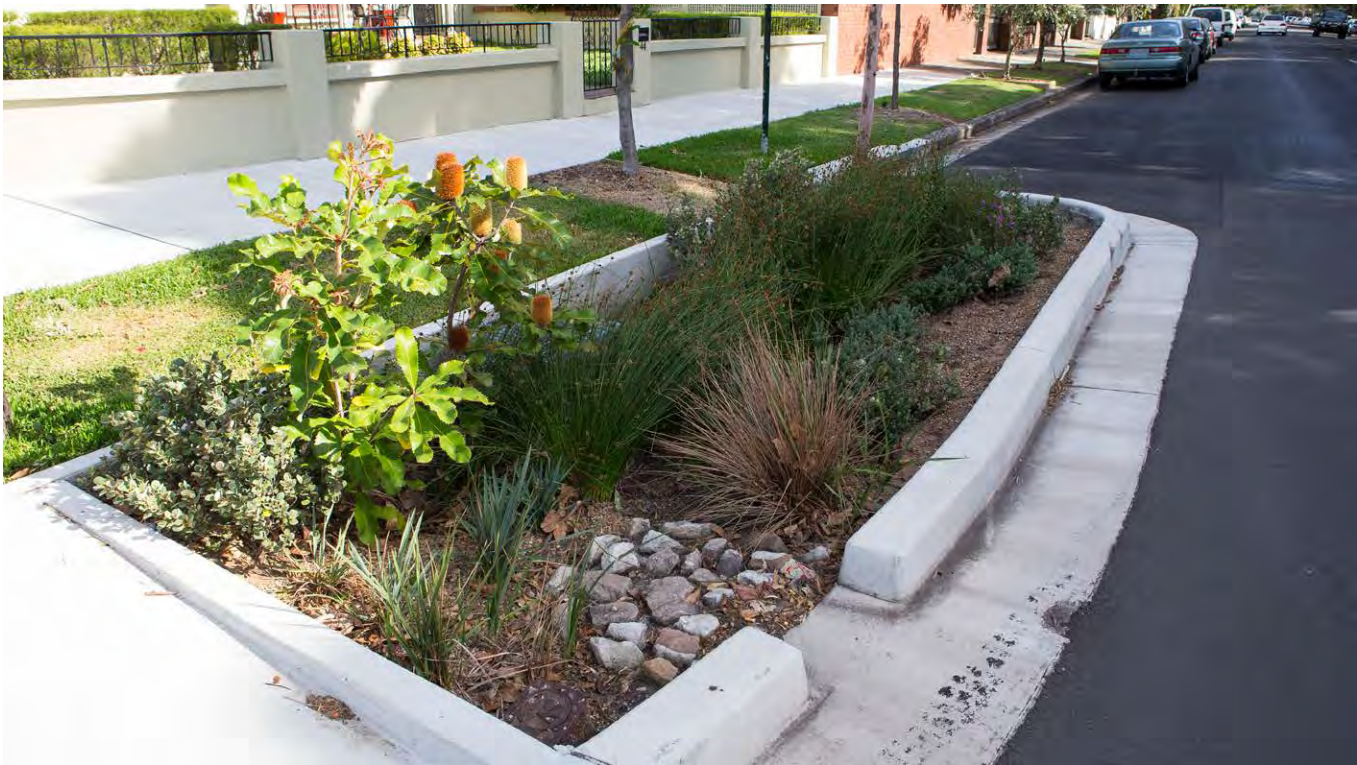
Example of existing corner build-outs with passive irrigation in the City of Sydney (image credit City of Sydney)
