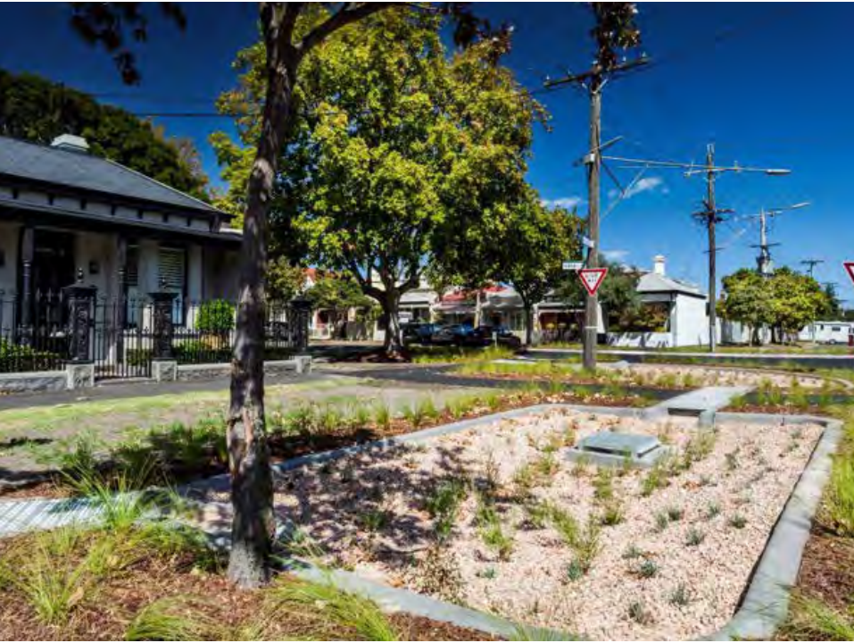
Figure 57: Rain garden in Park Road, Middle Park (Source: City of Port Phillip)
