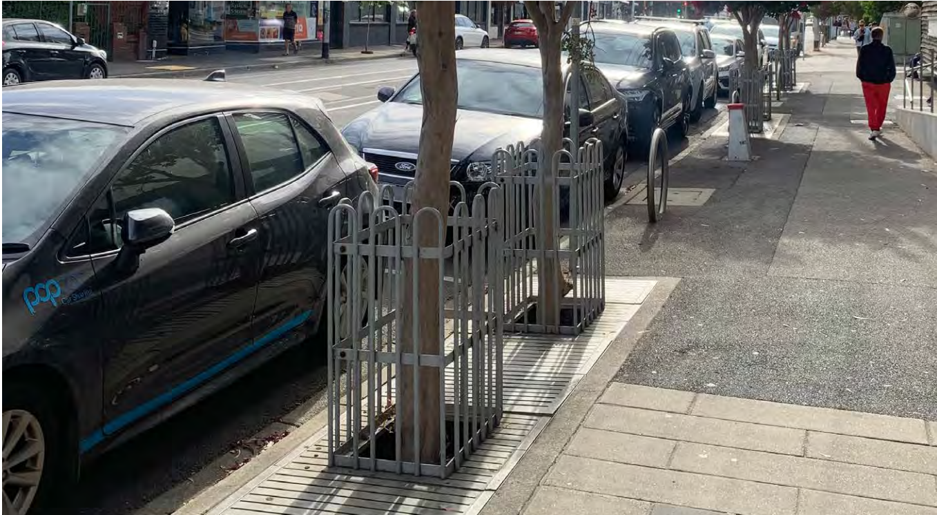
An example of tree cut outs with trees planted into pits large enough for connected soil between pairings.
