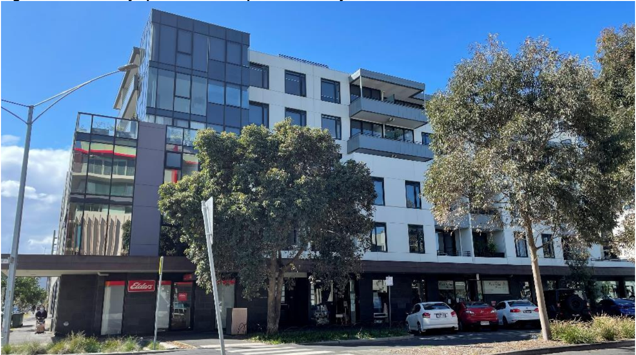
Figure 10 – Six storey apartment development at 55 Bay Street
