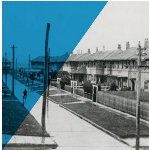
First houses built at Fishermans Bend sponsored by State Savings Bank of Victoria, 1930-1939. Port Phillip City Collection
