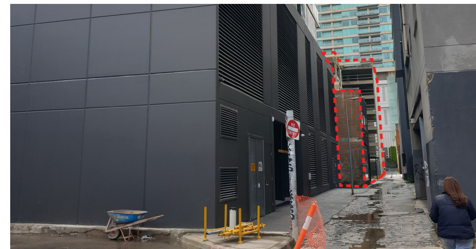
6. View of Site West from Little Bank Street
