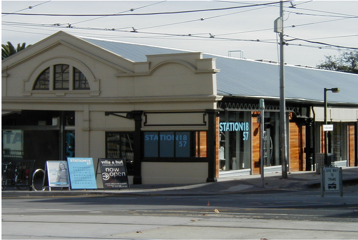
Photograph 1 – Former St Kilda Station building – Fitzroy St and St Kilda Light Rail line elevations.
