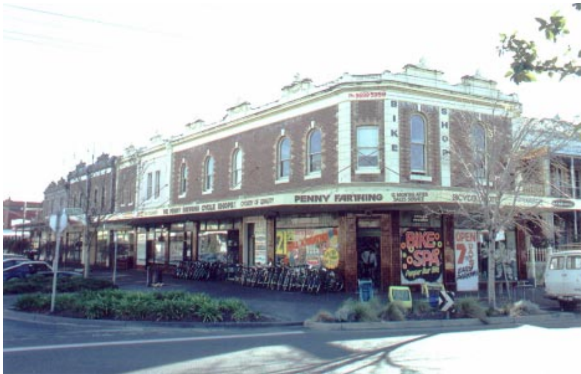
The Armstrong Street shops, Middle Park.
