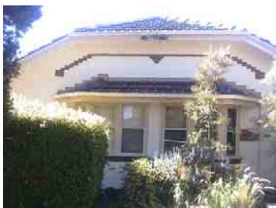
Unique gambrel-roofed house at 4-6 McCrae Street; note canted bay window across both dwellings
