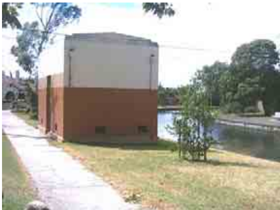
Bend in the canal at Goldsmith Street; note 1920s electrical substation on north bank
