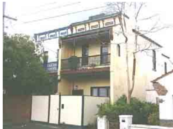
Atypical pair of rendered Victorian double-storey terrace houses at 15-17 Byron Street
