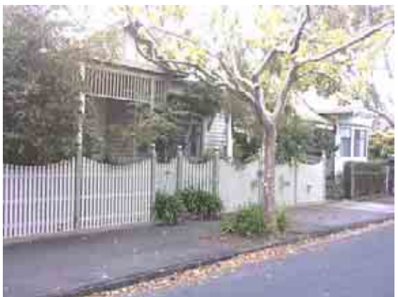
Row of 1910s detached weatherboard cottages on north side of Lawson Street
