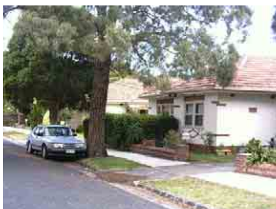
General view along west side of McCrae Street; note bluestone kerbing and street trees
