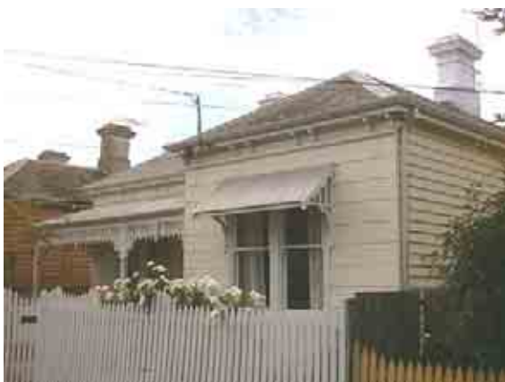
Typical double-fronted timber villa, one of several in a row in Moore Street
