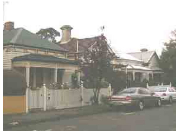
Row of detached single-fronted Victorian timber cottages in Mason Avenue
