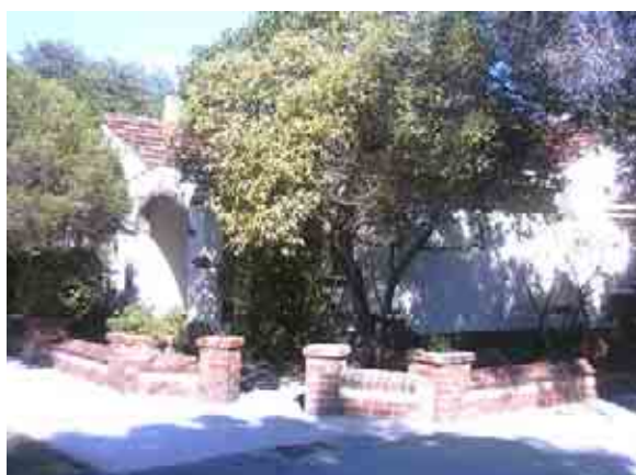
Tudor Revival-influenced house on corner of McCrae and John Street; note front fence
