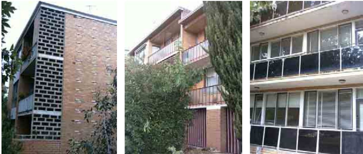
Figure 16 A selection of fine architect-designed post-war apartment blocks in Elwood (source: photographs by Heritage Alliance, 2005)
