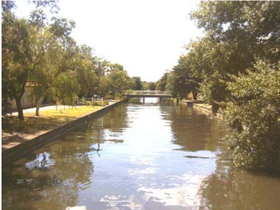
General view of the Elwood Canal; photograph taken after flood rains
