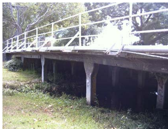
Reinforced concrete girder bridge at St Kilda Street, designed by John Monash
