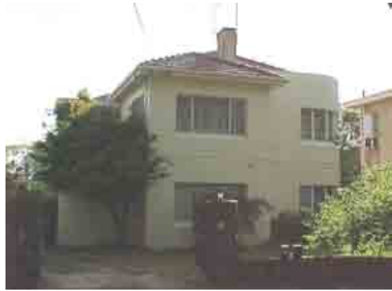
Figure 22 Flats, No 1 Holroyd Crt (c.1938)
