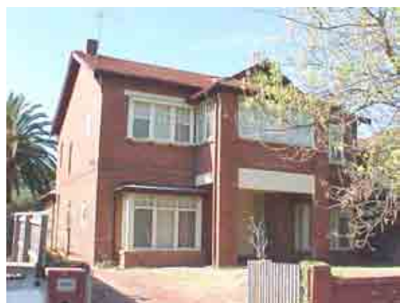
Figure 48 Wittonia Flats at No 27 (c.1922)
