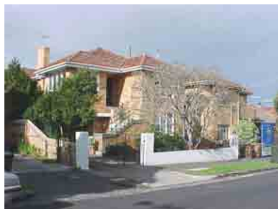
Figure 19 Double-storey flats at Nos 4 and 6
