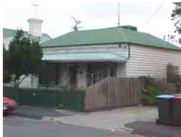
Figure 5 Double-fronted house at No 25
