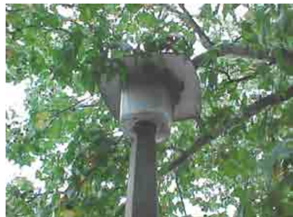
Figure 37 Detail of 1920s concrete lamp
