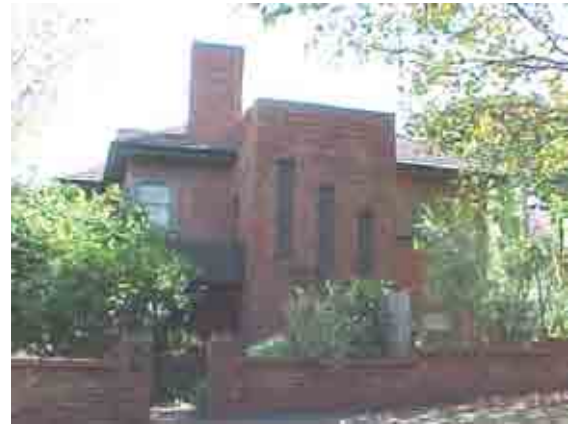
Figure 42 Flats, 18 Murchison Street (1938)
