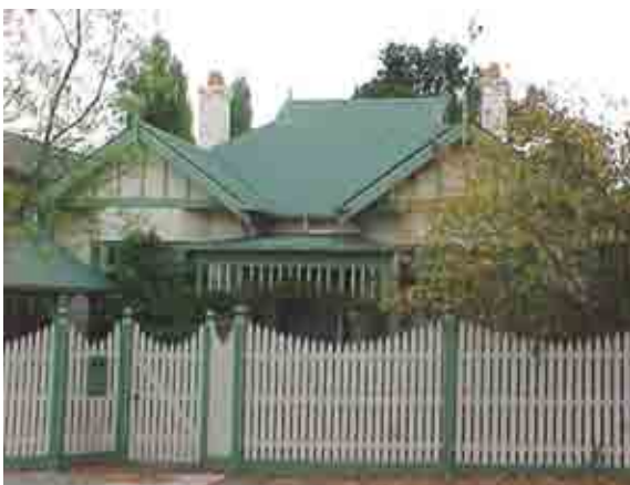
Figure 31 Weatherboard house at No 27
