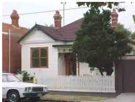
Figure 9 Weatherboard house at No 2
