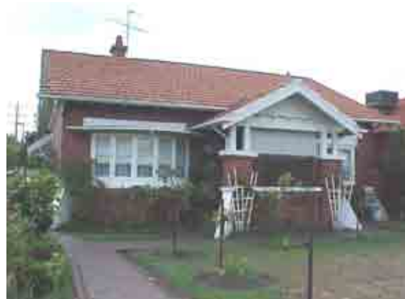
Figure 40 Bungalow, 160 Alma Road (c.1925)
