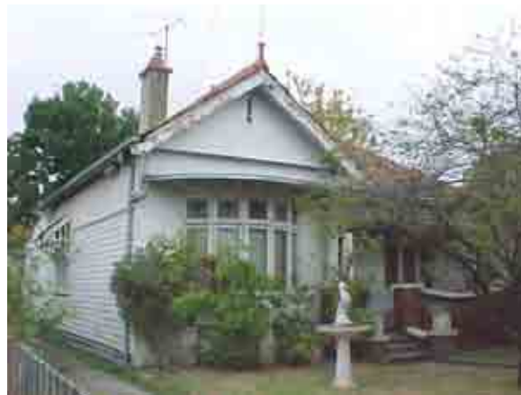
Figure 30 Weatherboard house at No 6
