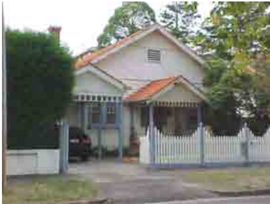
Figure 39 Timber house, 6 Murchison Street
