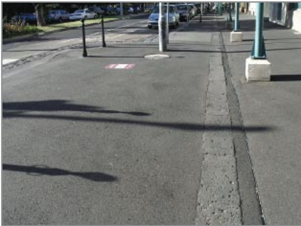
Photo 14. Bay Street widening Port Melbourne with bluestone kerb retained indicating the original road alignment
