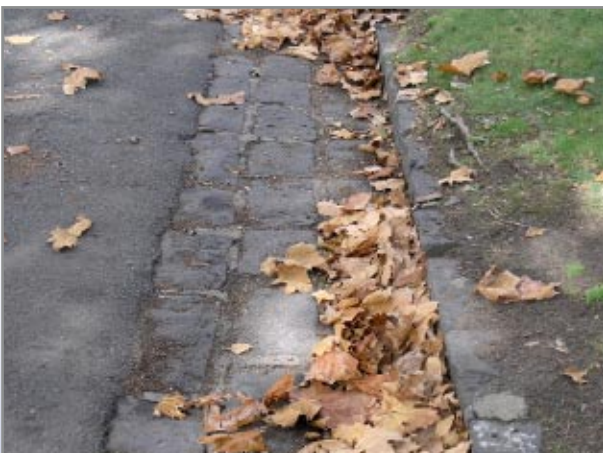
Photo 9. Shelley Street, Elwood
