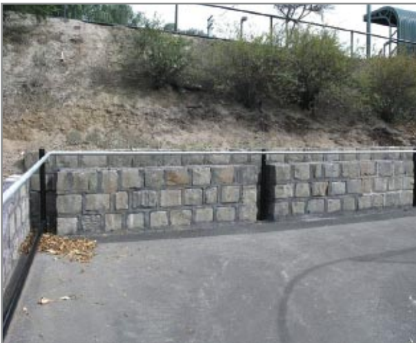
Photo 30. Retaining wall in Whiteman Street, South Melbourne
