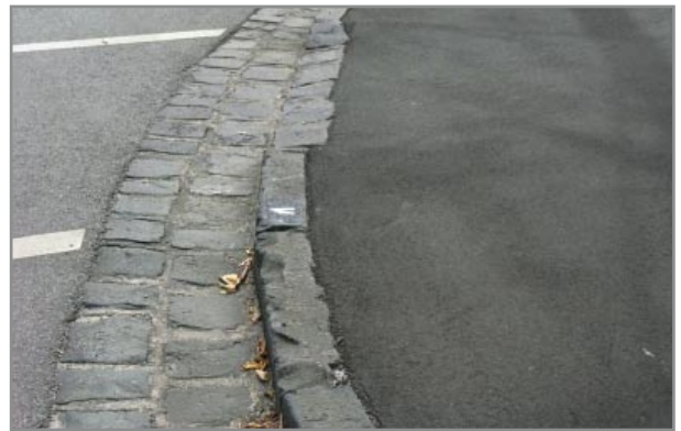
Photo 16. Corner Park & Cecil, more recent use of bluestone kerb and channel
