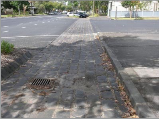
Photo 1. Cecil Street, South Melbourne
