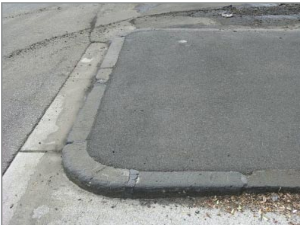
Photo 15. Douglas Street, South Melbourne
