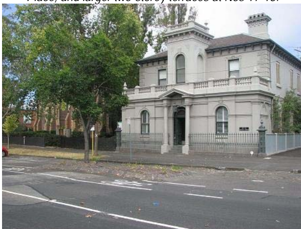
Figure 20 Former doctor's townhouse (later RAI A offices) at 30 Howe Crescent, with polychrome church alongside
