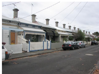
Figure 8: Row of single-fronted Victorian timber cottages, Erskine Street
