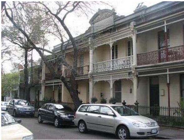
Figure 12 Suo Marte Terrace (1885), a fine row of double-storey rendered terraced houses in Ward Street
