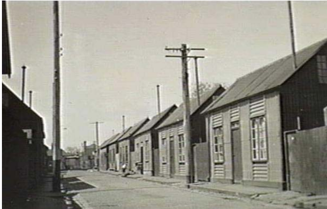
Figure 3 Robert Patterson's two-roomed prefabricated iron cottages in Patterson Place, still intact in a photograph taken in 1933 (source: Picture Collection, State Library of Victoria)
