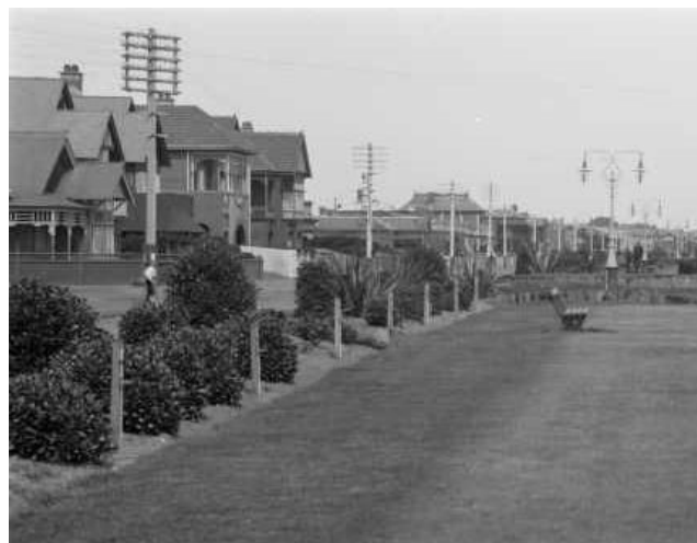
Figure 6: Early twentieth century postcard showing residential development along Beaconsfield Parade (source: Picture Collection, State Library of Victoria)
