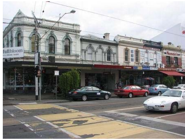
Figure 13 Row of ornate Boom-style rendered brick residential shops along Clarendon Street
