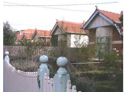
Figure 15: Row of Edwardian red brick villas in Ruskin Street, Elwood
