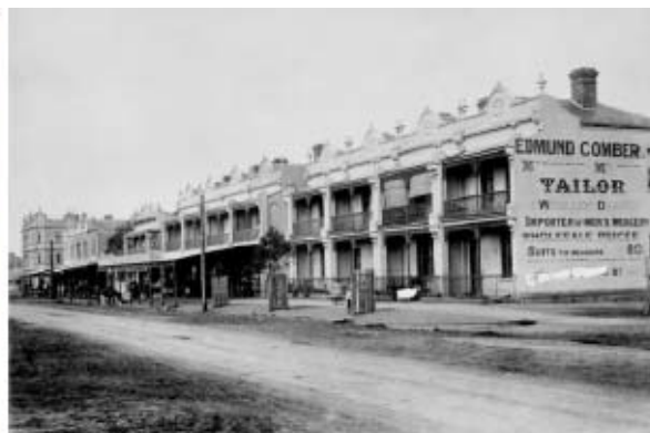
Figure 26 Terrace House, Victoria Avenue, Albert Park, 1889 (source: Port Phillip City Collection)
