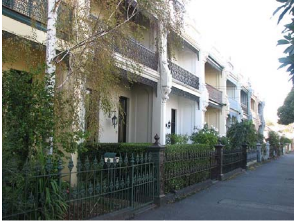
Figure 29 A particularly fine row of double-storey rendered terrace houses in Montague Street
