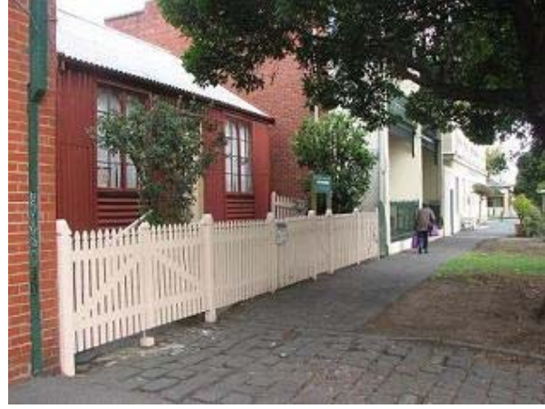
Figure 9 Prefabricated iron house (c.1853) at 399 Coventry Street, with double-storey terraces and corner hotel
