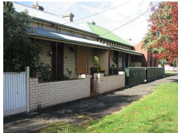
Figure 28 Double-fronted timber villas along Pickles Street. The low brick fence is not considered sympathetic.
