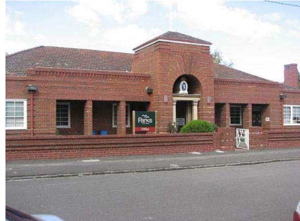
Figure 57 The former military drill hall (1935), on the park's northern edge
