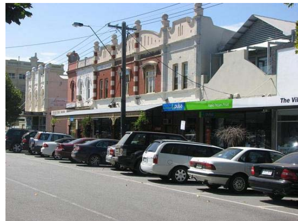
Figure 44 The mixture of Victorian, Edwardian and Inter-war Shops along the south of Armstrong Street
