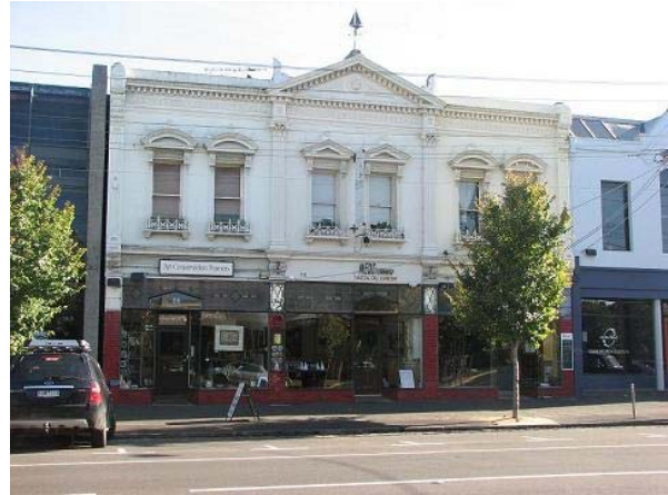
Figure 36 Group of three residential shops in Bridport Street, showing original shopfronts at ground floor
