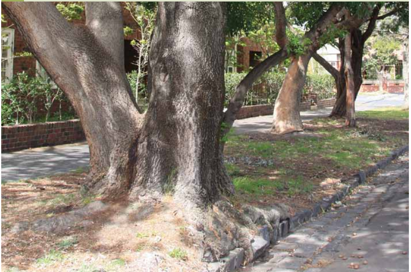
The roots of the mature Banksia breaking up the curb
