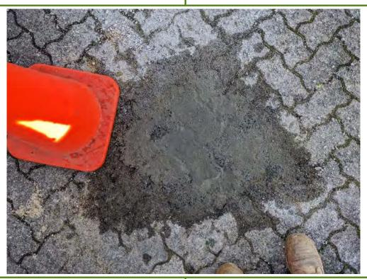
**Photo ID: 8** – Reinstated concrete in car park (SB05).
