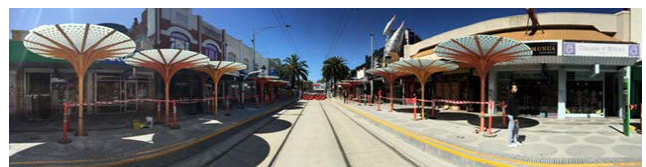
The new look Acland Street nearing completion.
