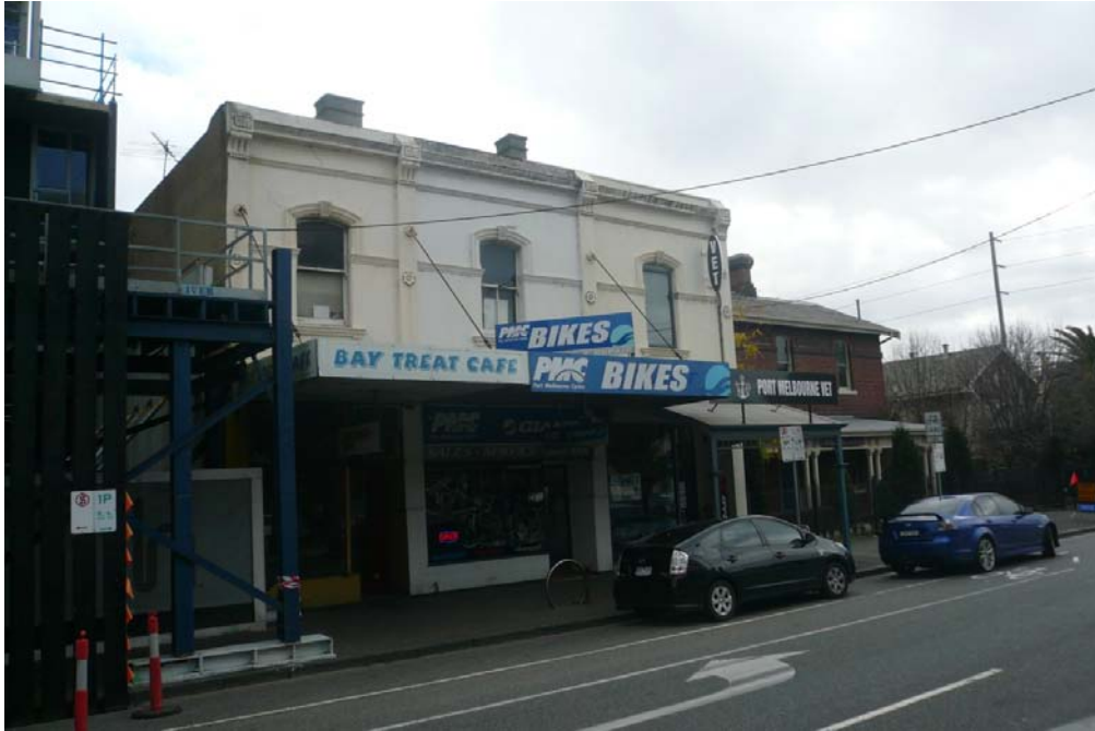
Figure 7 105-109 Bay Street and 113-119 Bay St, proposed to be retained within HO1
