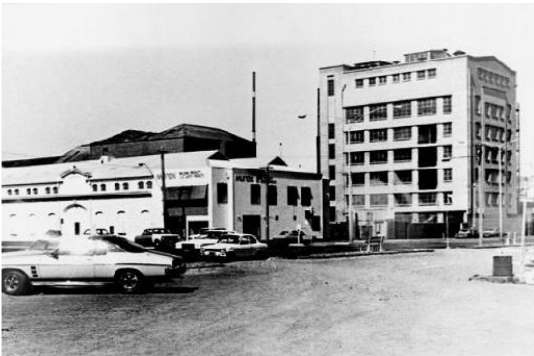
Figure 2 The Coal Depot photographed in 1975, showing the appearance of the building to Beach Street, subsequently altered. Source: City of Port Phillip Heritage Collection.
