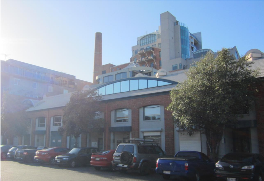
Figure 6 11 Beach Street showing elevation to Dow Street, looking east. This former single-storey warehouse building has been converted to a commercial use.
