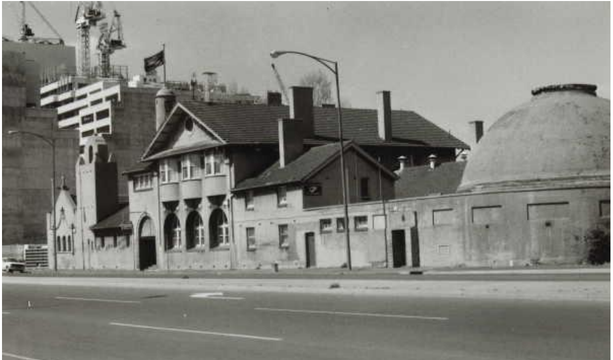
Figure 2 The former Anglican Missions to Seamen, now the Mission to Seafarers (1917), Flinders Street extension, Docklands, photographed in 1981. Source: John T Collins collection, State Library of Victoria.
