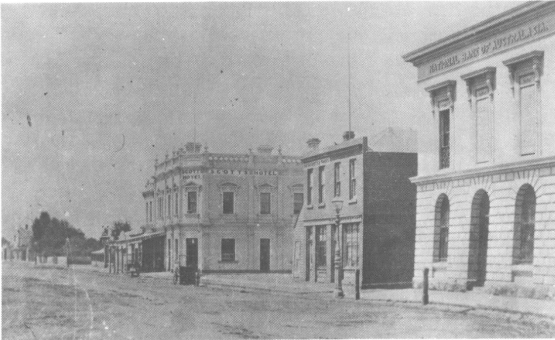
Figure 1 Bay Street, Port Melbourne c. 1878-79. The subject property is at the centre of the image.
