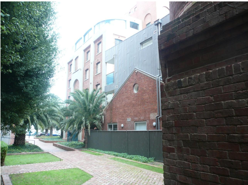
Figure 7 Looking south to Beach Street from the base of the chimney. The taller building in the background is Block 4. The 2009 zinc-clad additions to 50 Dow Street are also visible.
