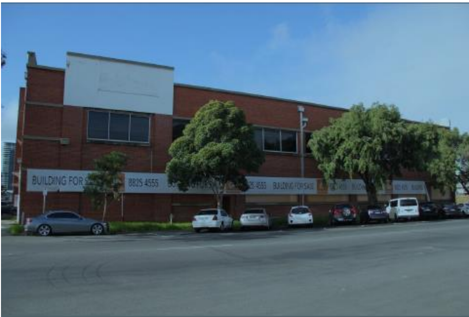
Former J. Kitchen building at 14 Woodruff Street
