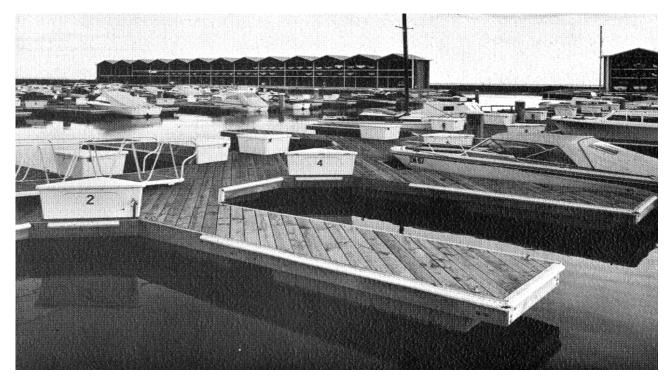
Figure 6: View of newly-completed marina, showing south dry boat storage building in background. Note floating berths, with diagonal timber decking, canted corners and triangular dock-boxes Source: <u>Wood World</u>, August 1969, p 13 (photographer uncredited)
