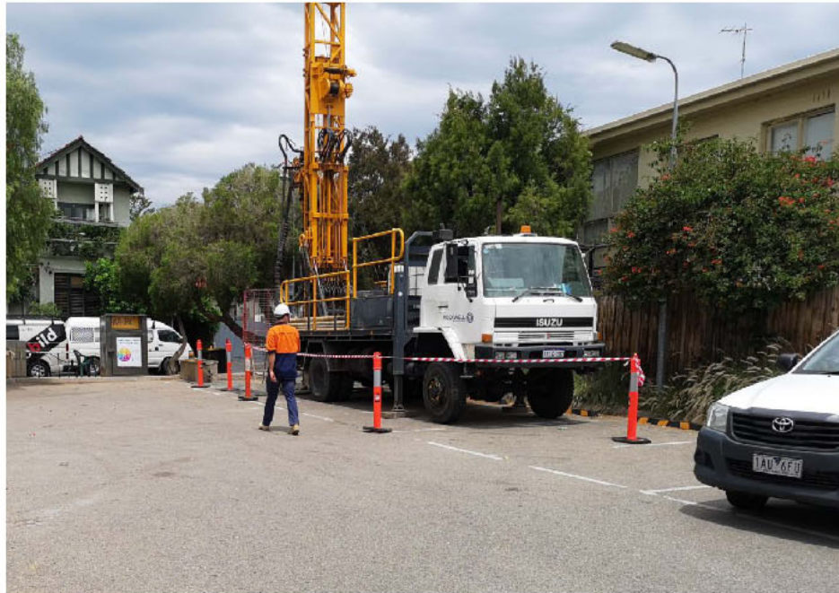
Photograph 1 : Drilling rig setup at borehole location BH01 (facing south)
