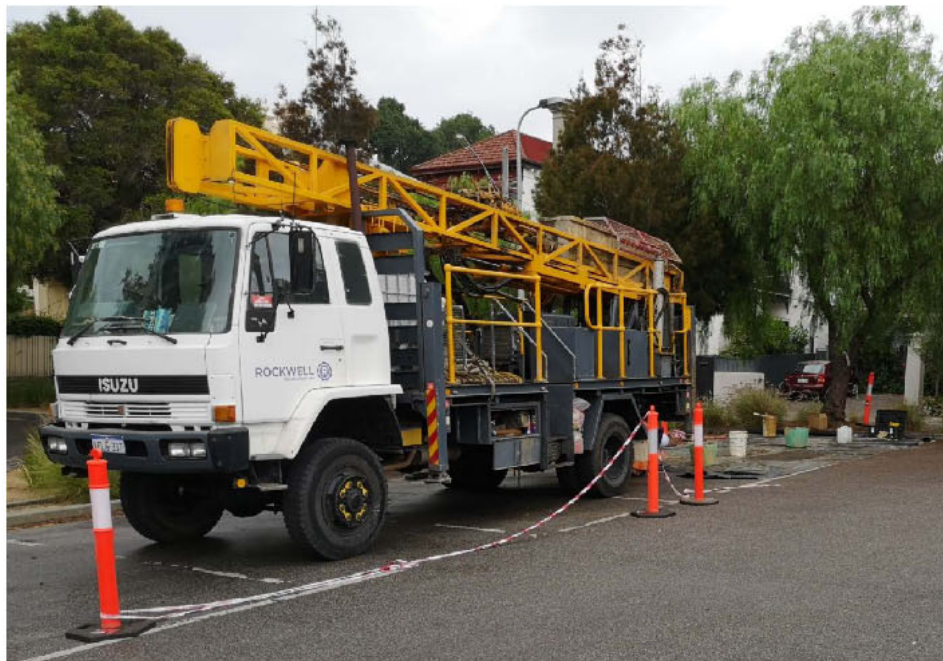
Photograph 2 : Drilling rig setup at borehole location BH03 (facing south east)
