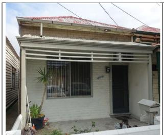
Figure 51. 279 Ross Street. Alterations: removal of chimneys, eaves brackets, verandah posts and ornament, reformatting front window, recladding in fake brick.
