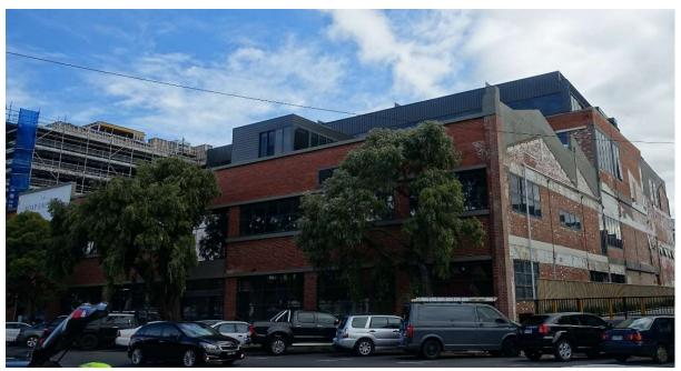
Figure 25. 14 Woodruff Street, following demolition of its southern neighbours. The profiles of the gabled and sawtooth roofs of the adjacent building(s) are visible on the south wall.
