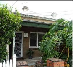
Figure 50. 269 Ross Street. Alterations: removal of eaves brackets and verandah, reformatting window opening, recladding façade in fake brick.
