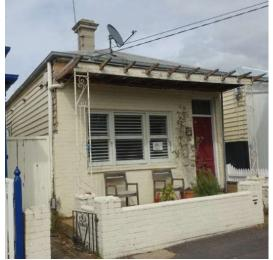
Figure 48. 133 Farrell Street. Alterations: removal of eaves brackets, verandah, reformating front window, and recladding front façade with cream brick.
