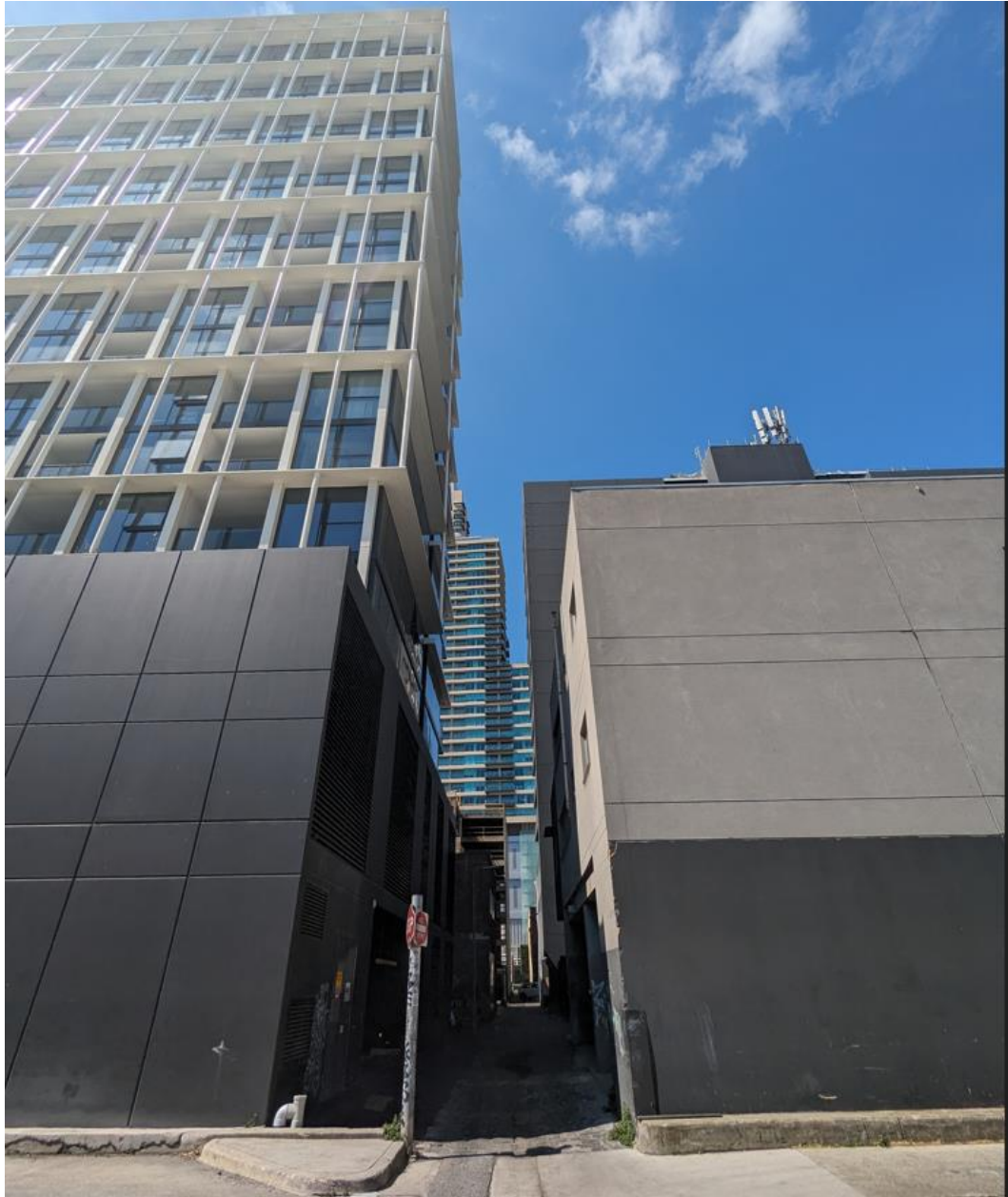
Figure 6 - Image viewing east along Little Bank Street from western extent (41-49 Bank Street visible front left)
