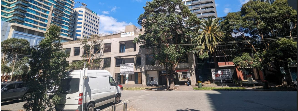
Figure 4 – Photograph of frontage of subject site as viewed from opposite side of Bank Street
