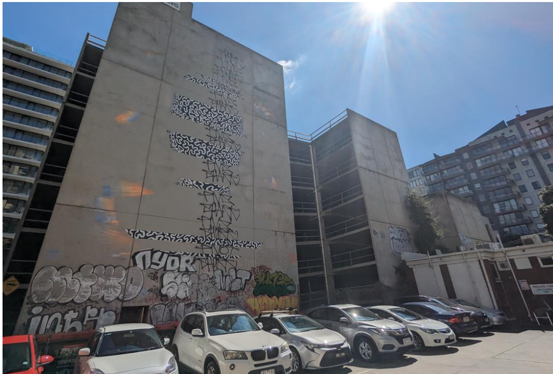
Figure 10 - Viewing west from rear carpark to subject site from 1 Bank Street
