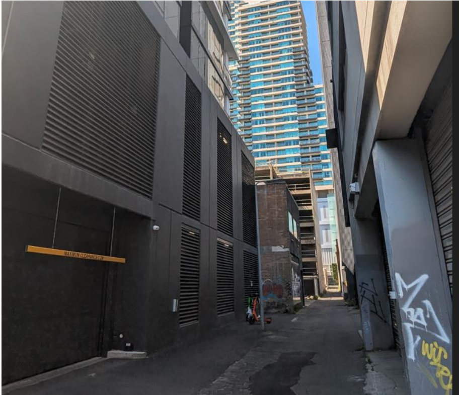
Figure 7 - Image viewing east along Little Bank Street, 41-49 Bank Street seen at left of image
