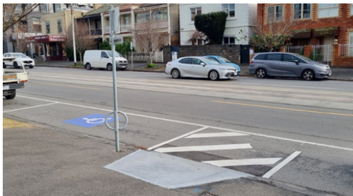
Park Street upgraded parking space.
