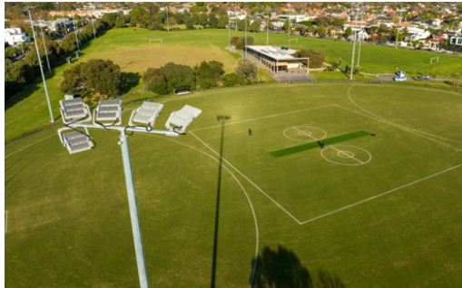
New lighting upgrade at Elwood Park.
