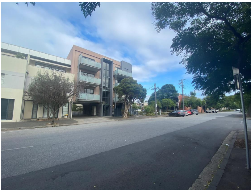
Photograph 17: Looking west, across Boundary Street, to apartment and townhouse development at No's 9-19 (three and four storeys in a General Residential Zone)
