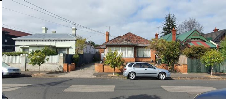
Figure 2 - The three sites that make up the development site. No's 21, 23, 25 The Avenue.
