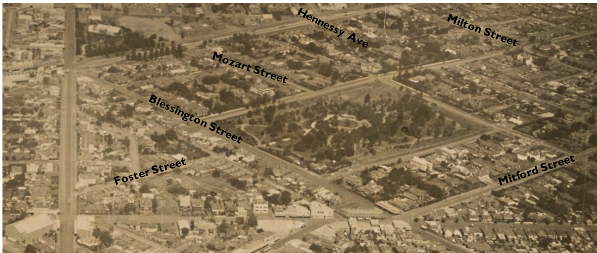
Figure 20 - 1924 aerial (SLV, E Ebell, H91.365/3)
