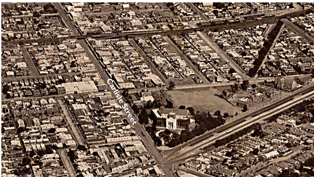
Figure 12 - Circa 1925 aerial – the portico of the Town Hall had been added (Source: SLV, 1920-30s 'ST Kilda TH -W R Garrett, H98.129-21)
