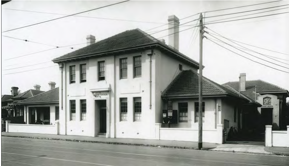
Figure 19 - Circa 1930 image of former Police Station and Court House on Chapel Street (Source: PPHC, sk0426)
