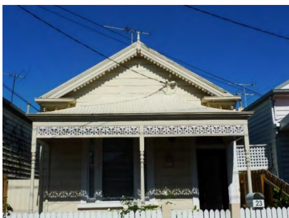
Figures 22 & 23 - 23 Brunning Street (left), broken bed gable with cast iron fringe, 19 Nightingale Street (right), typical Victorian period rendered chimney
