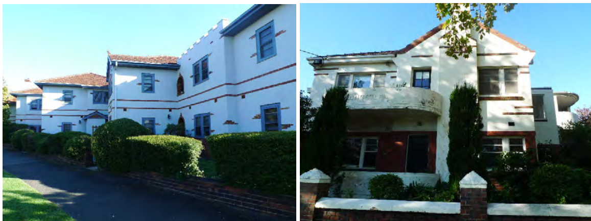
Figures 36 & 37 – Milverton , 22 Glen Eira Road (left) and Brightlea , 98 Brighton Road (right)
