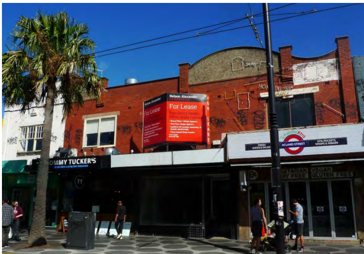
Figure 28 - 139-145 Acland Street, early 1920s with some Arts and Crafts elements
