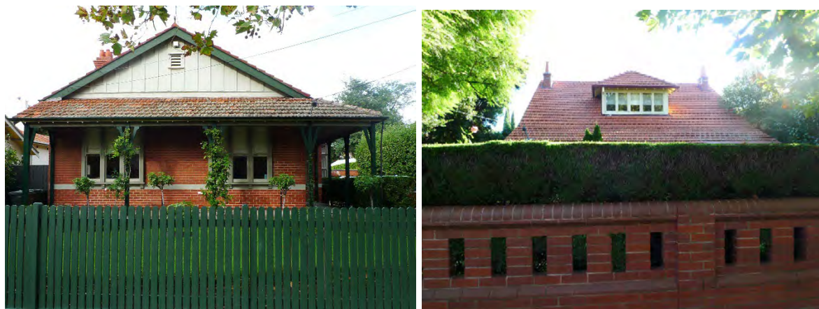
Figures 29 & 30 - 10A Quat Quatta Avenue (left) and 4 Erindale Avenue (right)
