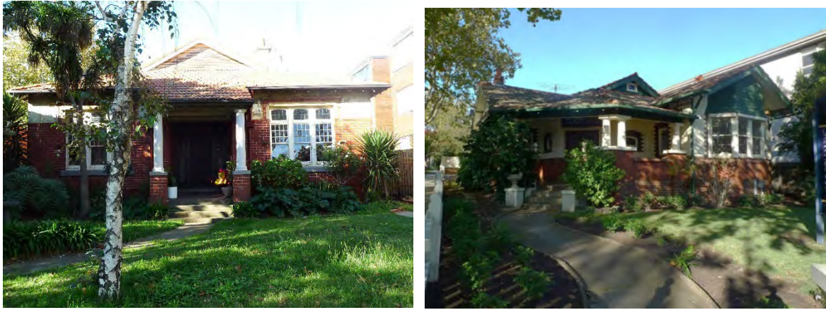
Figures 27 & 28 - 86 Brighton Road (left) and 100 Brighton Road (right)
