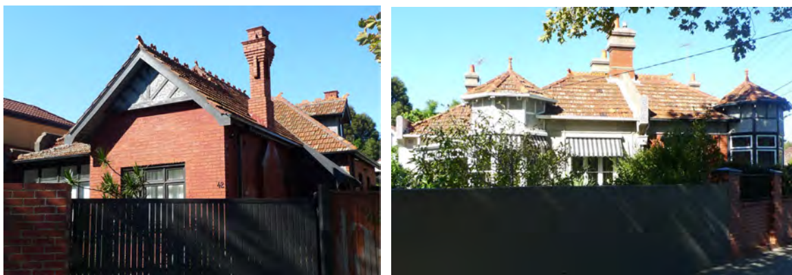
Figures 12 & 13 - 42 Brighton Road (left), 44 and 46 Brighton Road (right)
