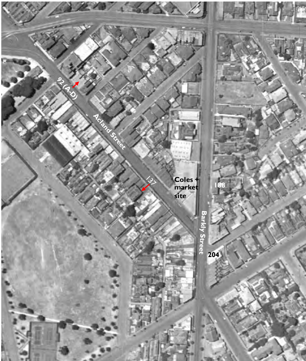
Figure 22 - 1945 aerial Project No. 5, Run 17E, Frame 58011 (Source: Landata)
