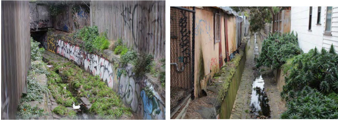
Figures 18 & 19 – section of early bluestone drain west of Lynott Street (left) and east of Lynott Street (right)
