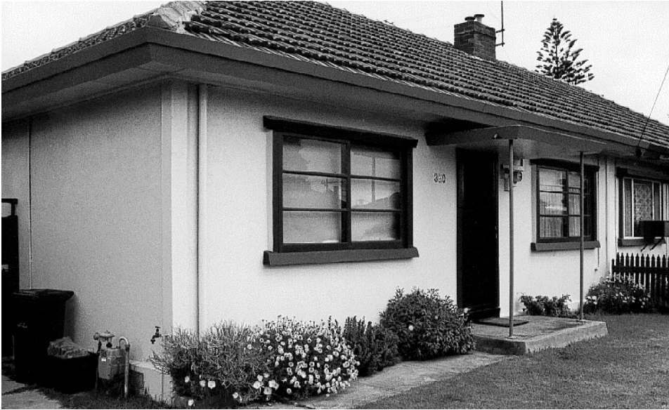
Figure 25. The original details of a concrete dwelling. Note the splayed eaves verge and splayed gutter, the eaves boxing, the partially concealed downpipe and the sliding timber windows with horizontal glazing bars set directly in the projecting concrete architrave in which the tracks are located.
