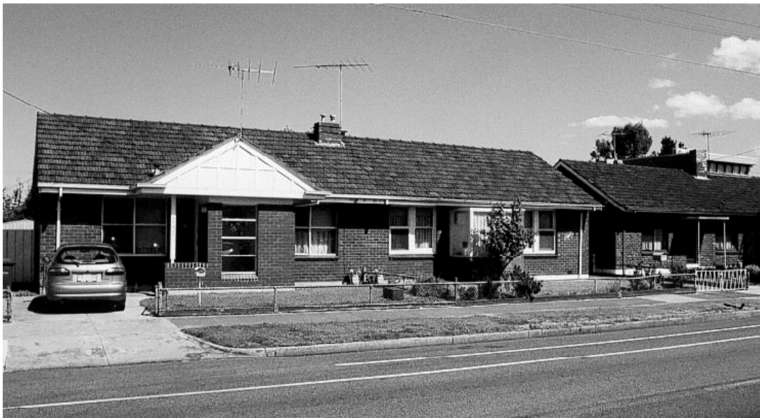
Figure 11. The dwelling to the left of the pair has an HCV porch and aluminium windows. That to the right has its original timber double hung windows and porch (now built in).
