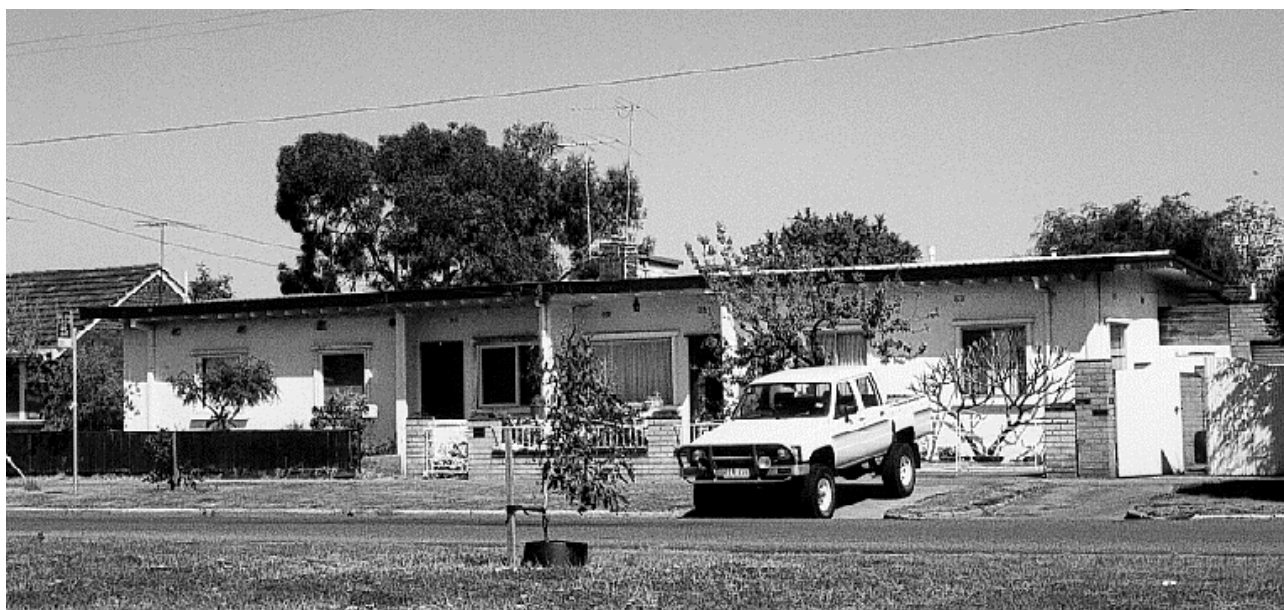
Figure 4 The first experimental dwellings using the TW Fowler system of concrete prefabrication, 324-326 Howe Parade, Fishermans Bend Estate.
