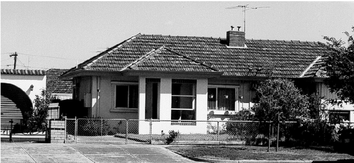
Figure 26. Later rendered brick porches on concrete dwellings.
