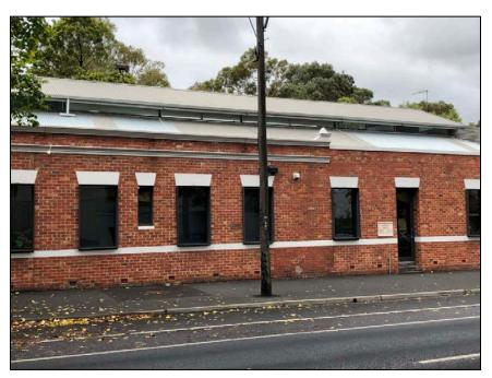
Figure 10 The Ferrars Street elevation of the subject building. The metal window shrouds and glazed windows are non-original. The two cornices that span the parapet of part of this elevation are of a modern segmented construction, suggesting they date from the same period as the window shrouds, ie they are not of traditional construction. The roof has been extended to form a first floor. The brick facade has been subject to extensive change.
