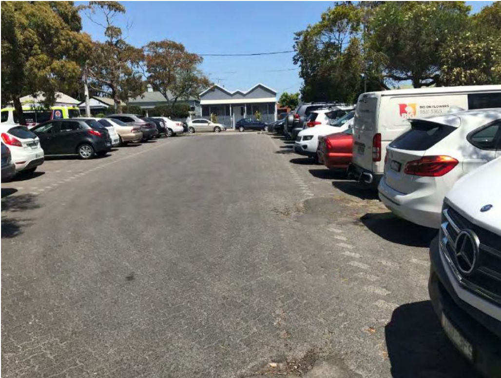
Photograph 1 – Facing south, Car park surface, 50 – 58 Marlborough Street, Balaclava
