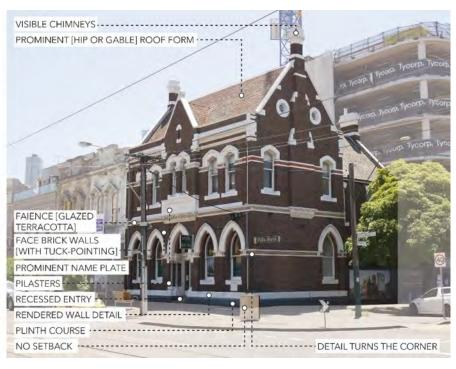
**Figure 35.** Large corner commercial building typology, showing typical features.
