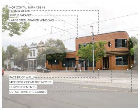
**Figure 33.** Corner commercial building typology, showing typical features.
