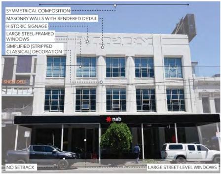
Figure 34. Large commercial building typology, showing typical features.
