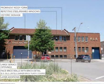
Figure 38. Industrial building typology, with visible roof form, showing typical features.
