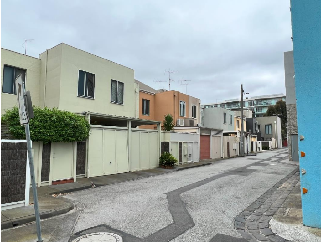
Figure 5: Rear interface of the Portview Square fronted properties, viewed from Donaldson Street
