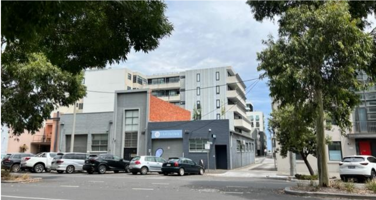
Figure 3: Photograph of frontage of the subject site as viewed from opposite side of Rouse Street
