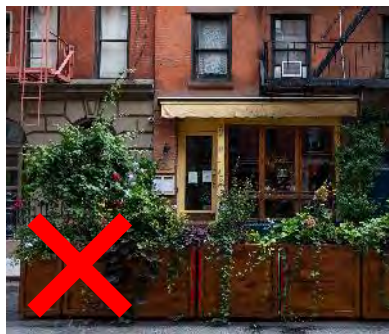
Figure 32: Planting is high and obstructs lines of sight.
