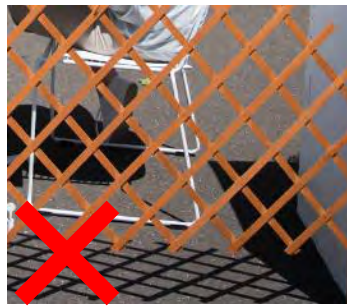
Figure 13: Flimsy materials like lattice should not be used.
