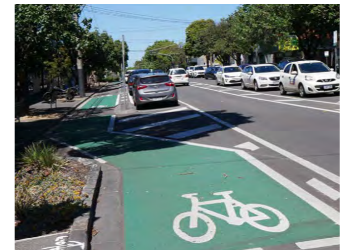
Image 79. Existing protected bike lane on Moray Street
