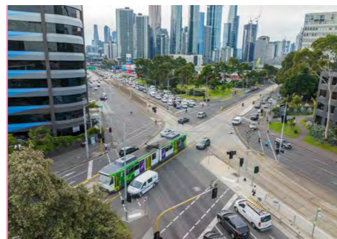
Image 65. Existing Kings Way and Dorcas Street junction aerial view
