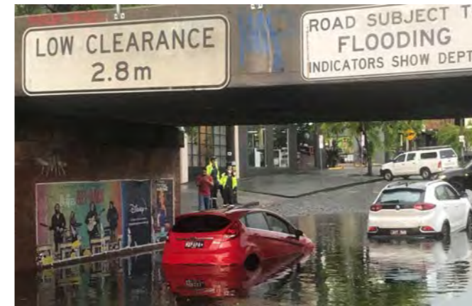
Image 37. Existing York Street underpass showing its flooding issue
