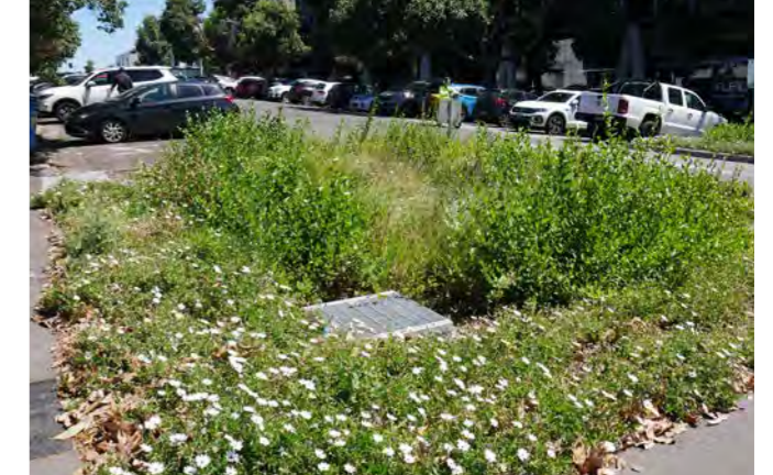
Image 38. Existing Market Street's WSUD initiative with kerb outstands
