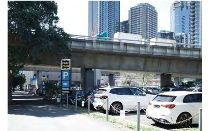
Image 51. Existing undercroft car park on Morray Street
