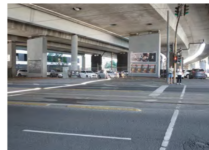
Image 69. Existing undercroft car park under West Gate freeway, East Clarendon Street
