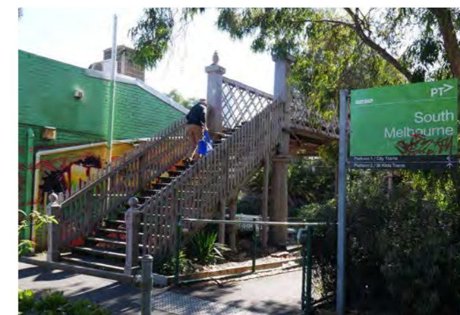
Image 73. Existing non-DDA-compliant footbridge viewed from Ferrars Street
