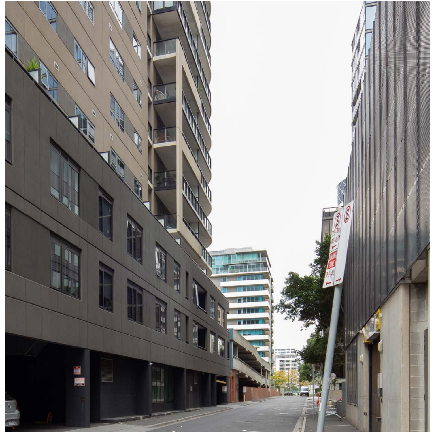
South Approach: Existing
