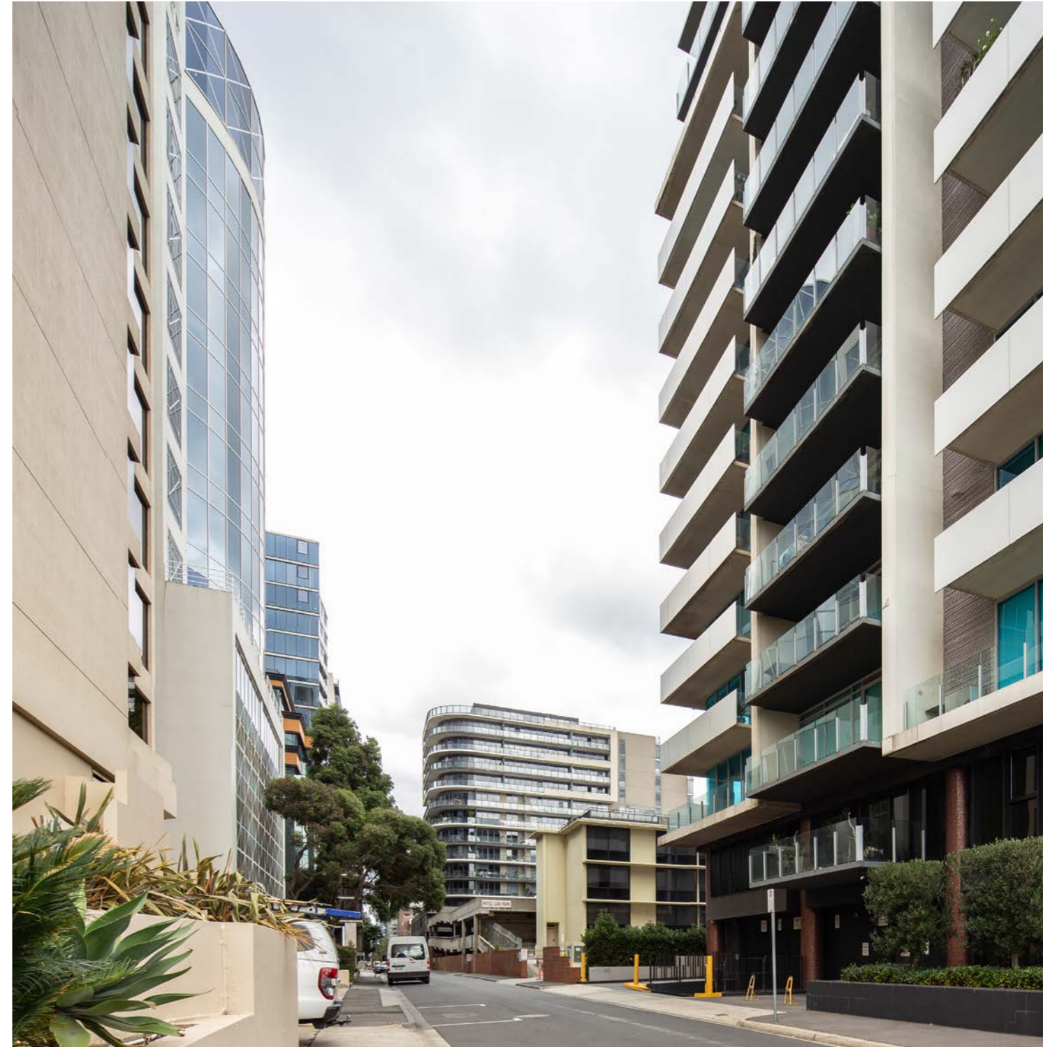
North Approach: Existing
