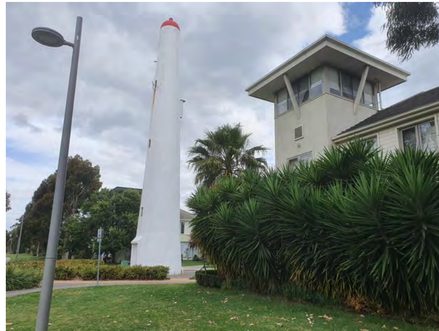
OBLIQUE VIEW OF SUBJECT SITE AND REAR LIGHT TOWER
