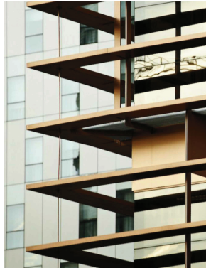
LVR01 Horizontal and vertical sun protection louvres, aluminium, anodised finish
