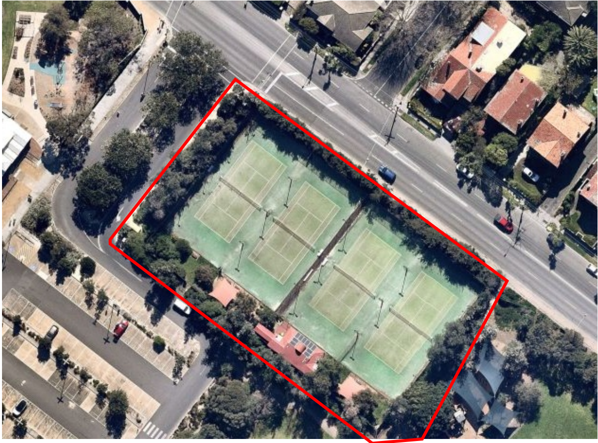
Figure 21 Tennis court and surrounding planting. Red line shows approximate curtilage
