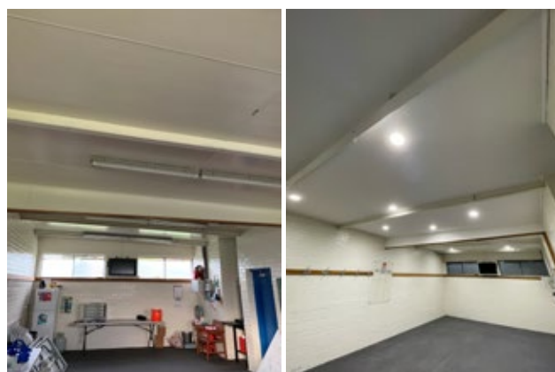
Pavilion Ceiling (Before)
