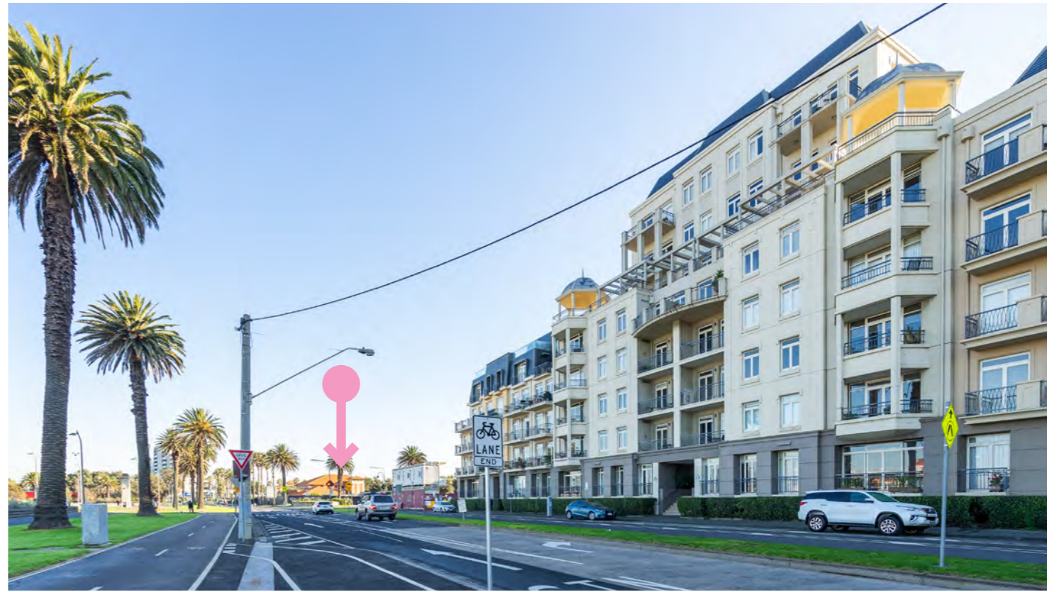
1 - BEACH STREET_ LOOKING WEST
