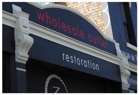
Showing different console bracket detailing - bracket on the left (single storey section), bracket on the right (two storey section).
