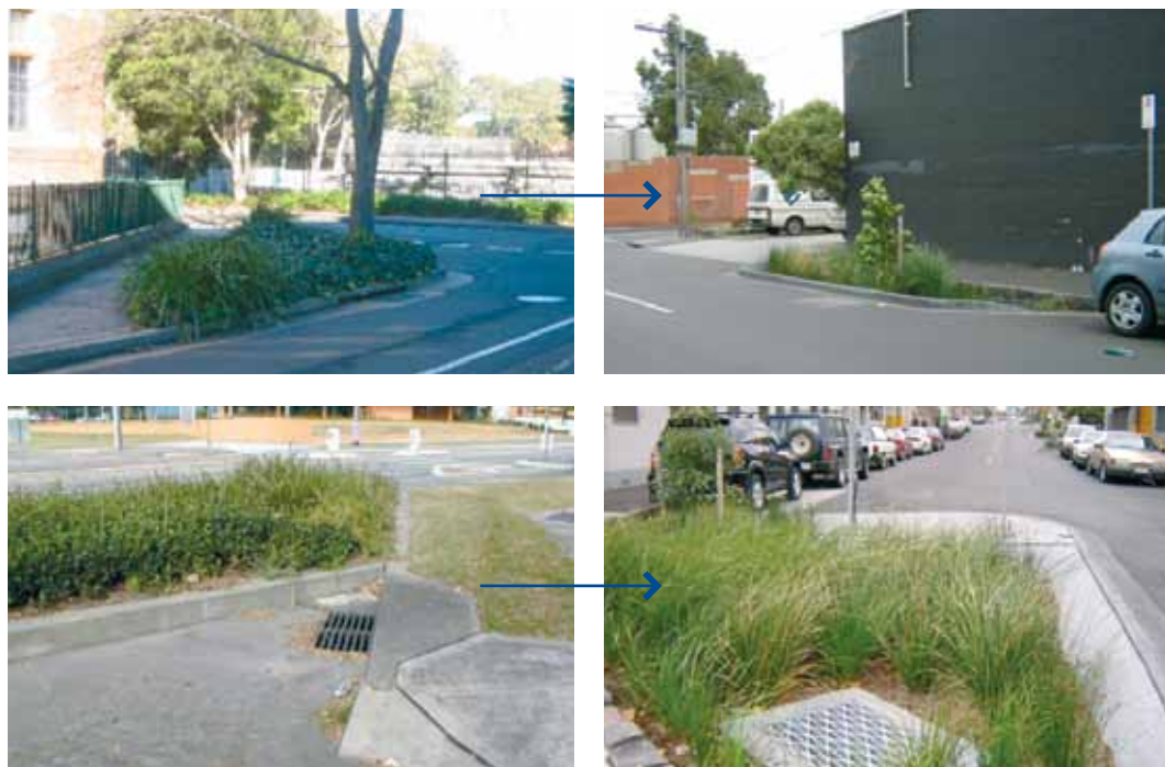
Figure 29. Medians and vegetated road verges can be retrofitted to accept stormwater for treatment.
