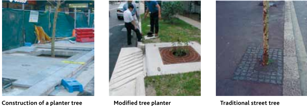
Figure 28. Street planter boxes showing the construction of a planter, a modified tree planter and a traditional planter box.
