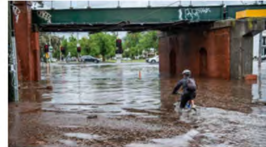
Cyclist at Montague Street Bridge during flooding event
